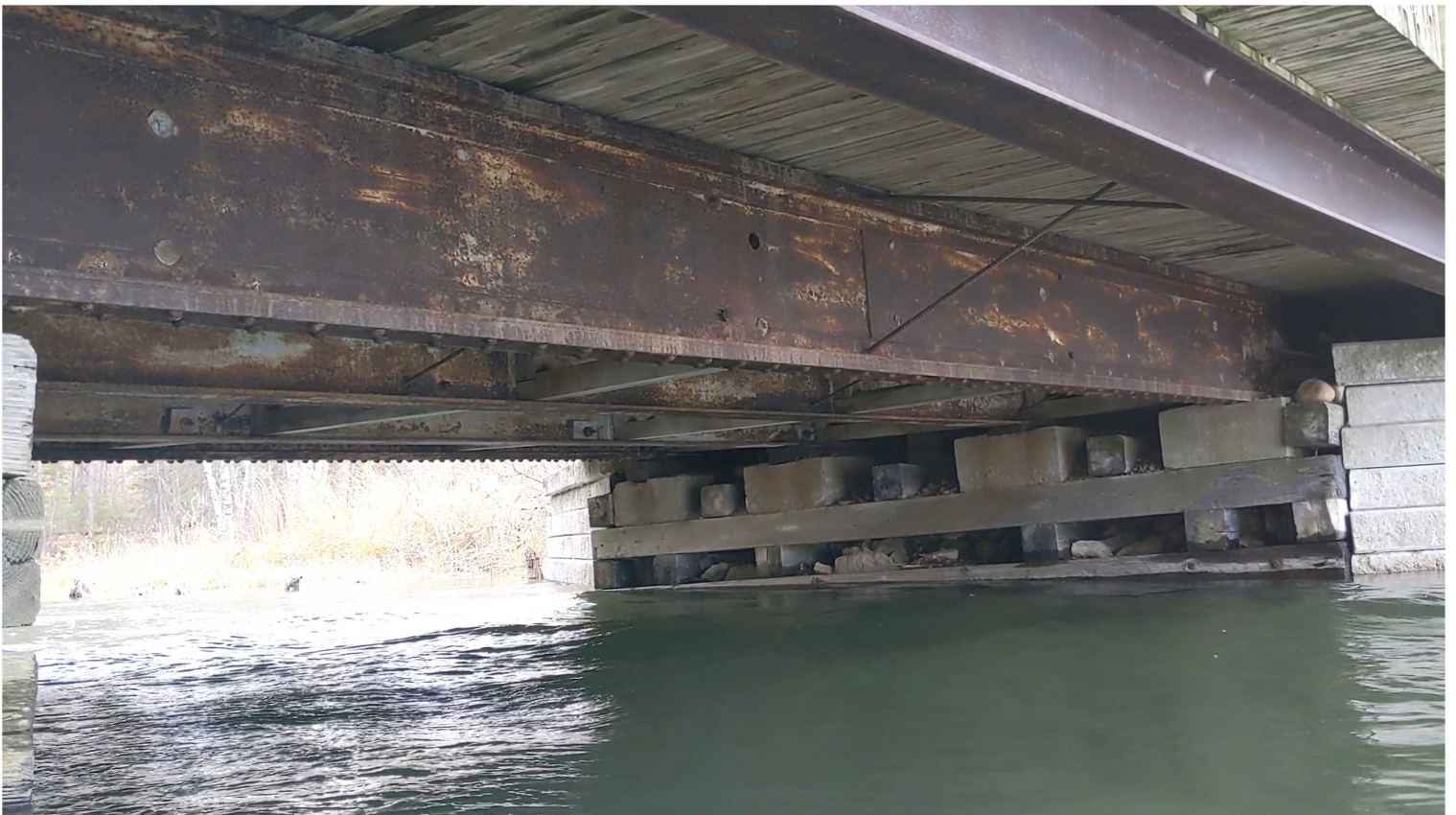
16. Interior Girder - See Corrosion (typ) (looking southwest)
