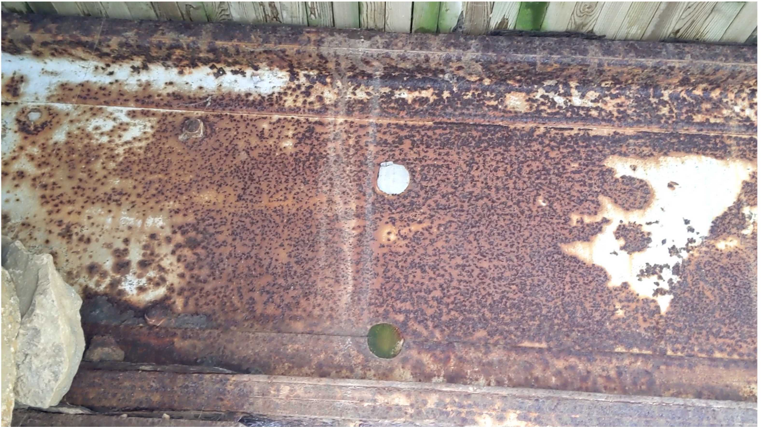
17. Heavy Corrosion at Ends of Girders (typ)
