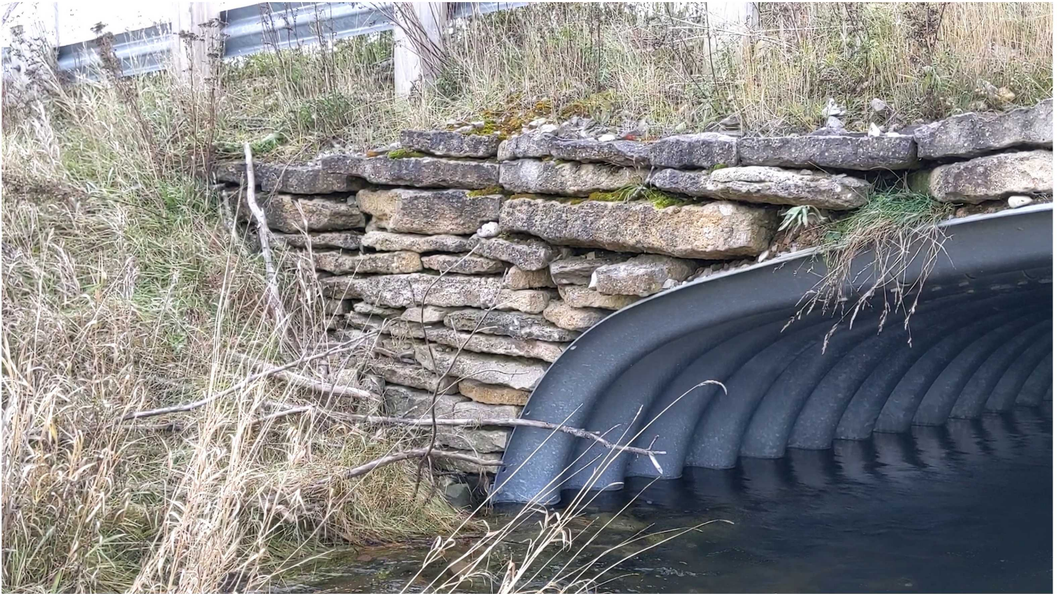
9. Retaining Fill at Northeast Corner - See voids (looking southeast)
