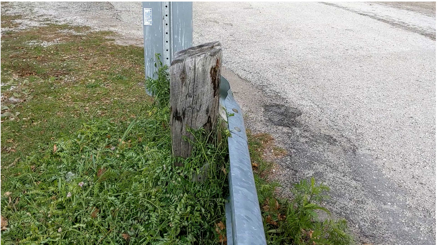
12. Rotten Post at Northeast Corner of Bridge
