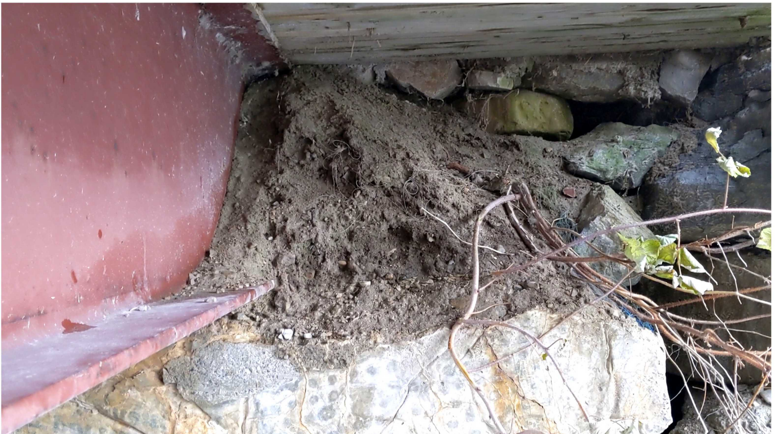
10. See Fill Below Deck - Caused by Lack of Ballast Wall at Corners
