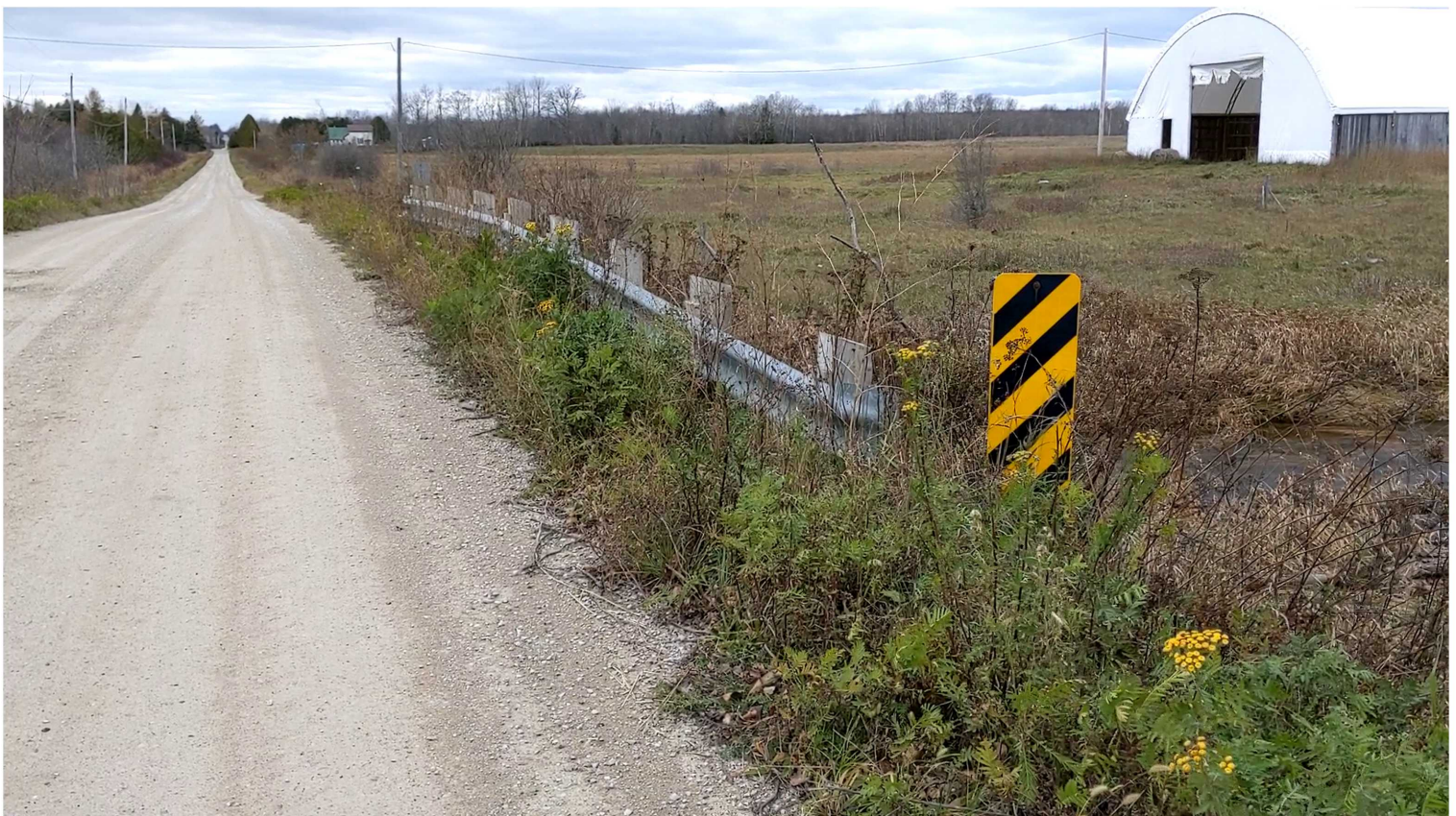
6. North Barrier (looking west) - Note barrier is too low
