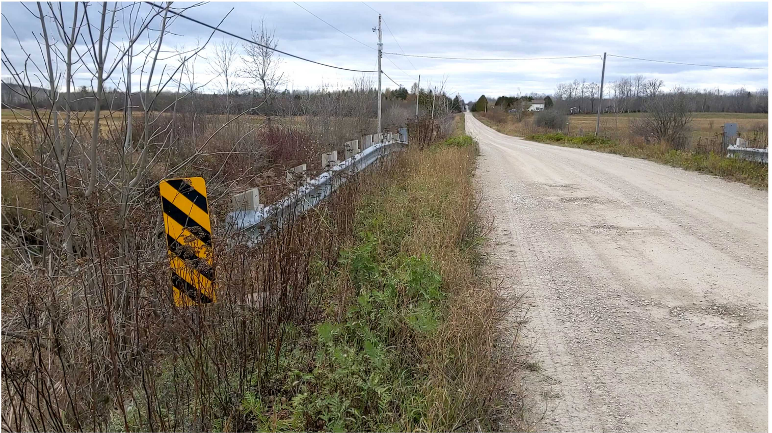
7. South Barrier (looking west) - Note barrier is too low
