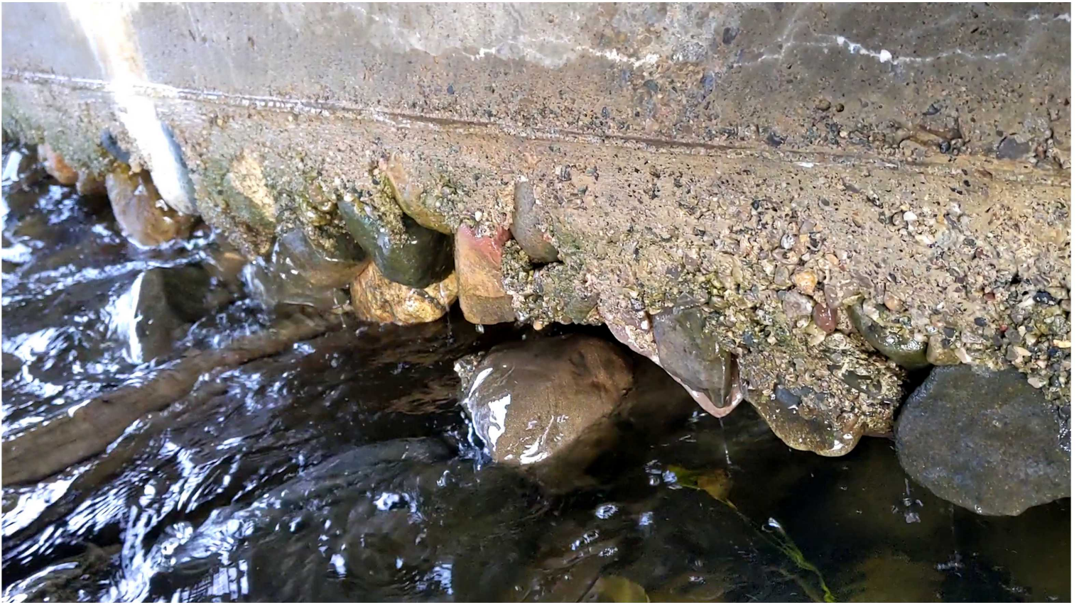
13. Bottom of East Abutment - Severely Undermined
