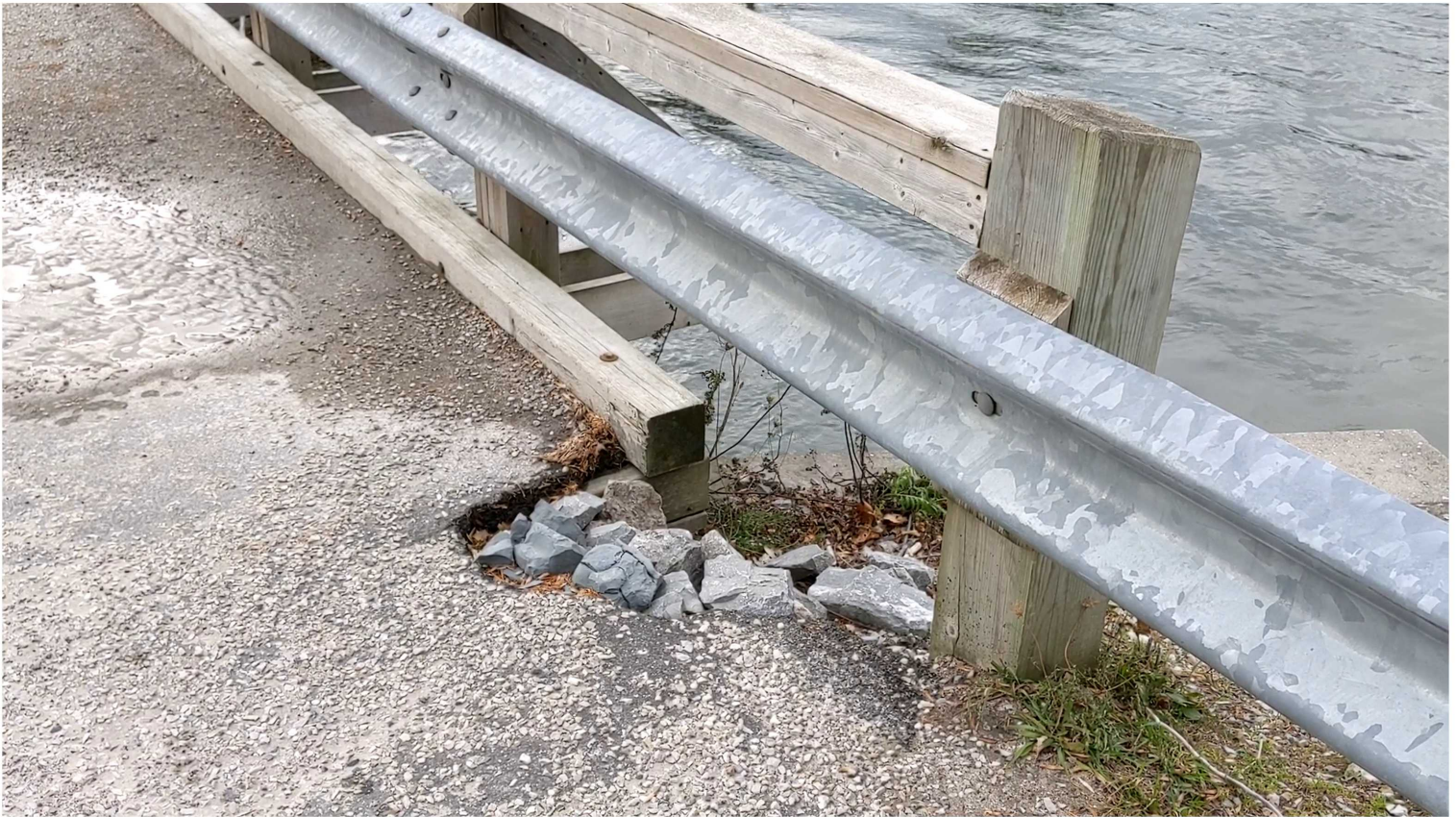
11. Erosion at Northeast Corner of Bridge (looking northwest)
