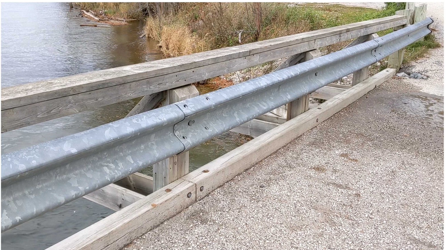
10. Barrier Panels Missing Bolts (typ) (looking northeast)
