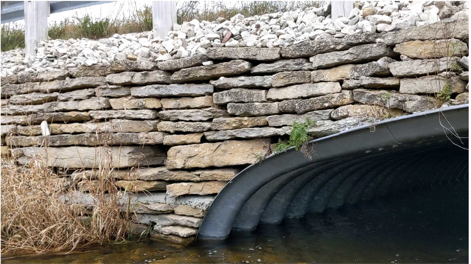
11. Retaining Fill at Southwest Corner - See voids (looking northwest)
