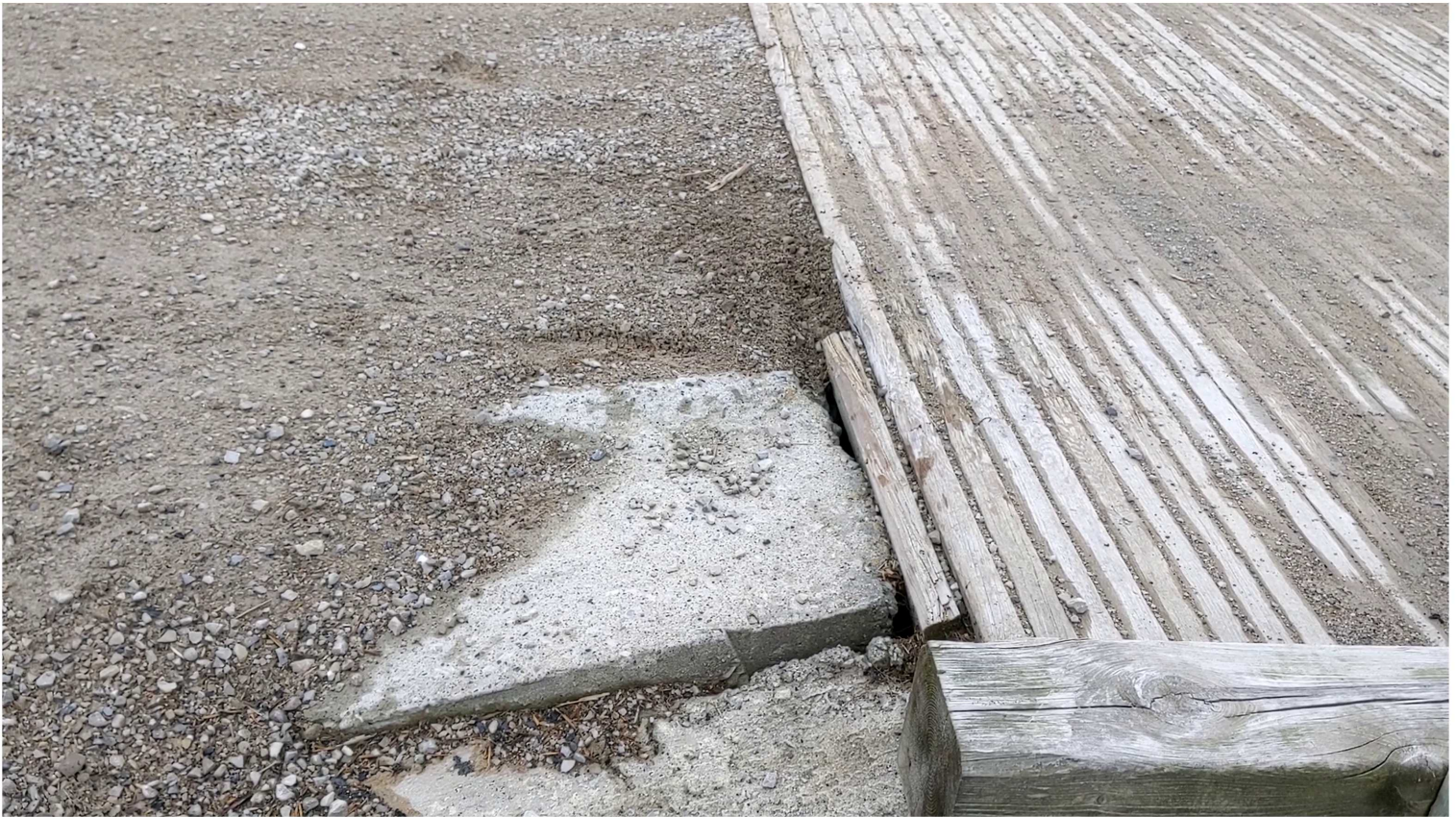
9. Erosion at Corners at Ends of Deck Due to Lack of Ballast Wall
