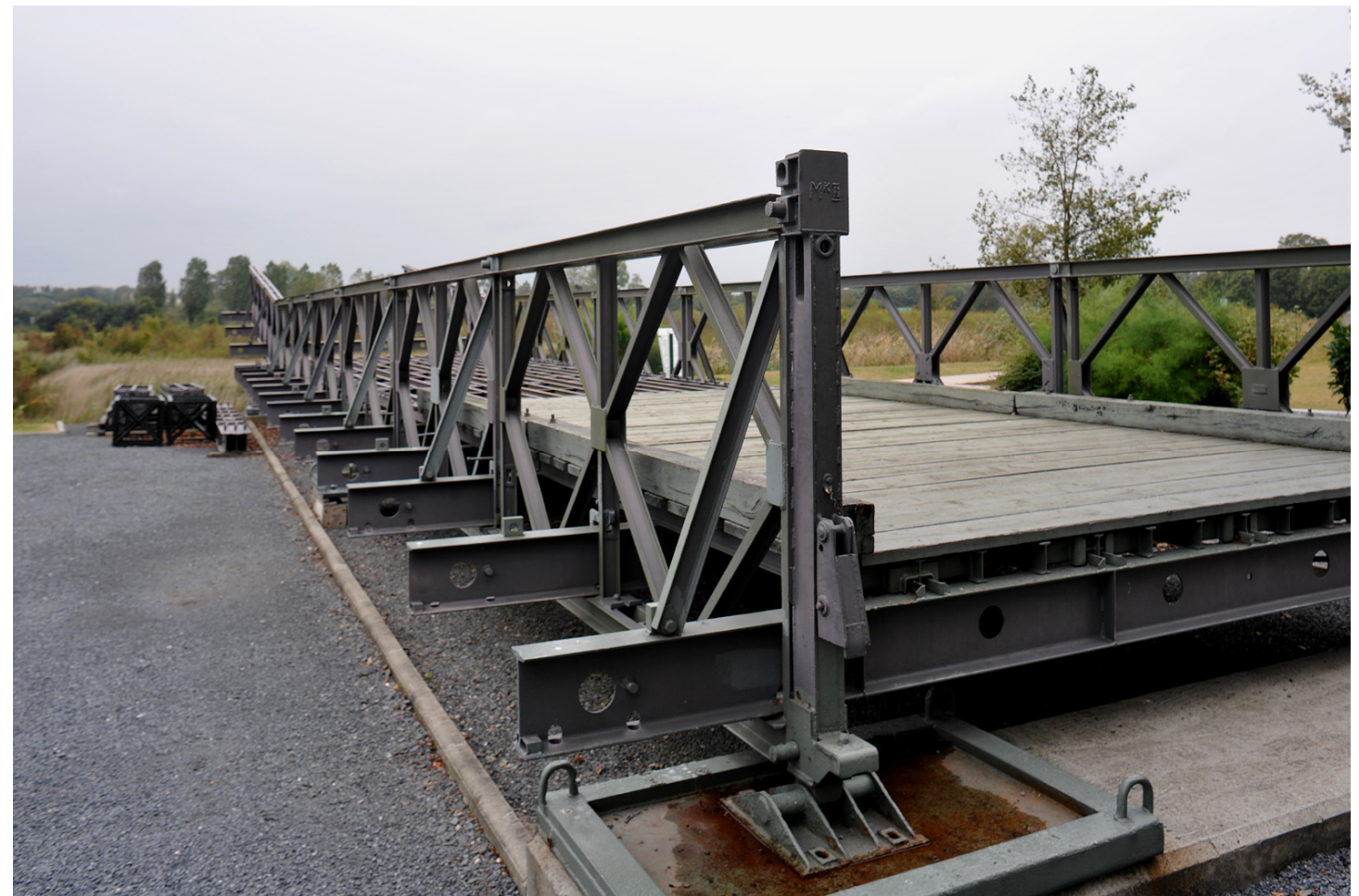
Bailey Bridge Example
